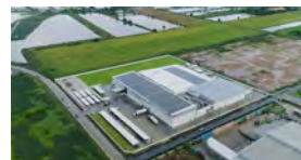
Solar power generation facilities (Thai Delmar Co., Ltd.)
