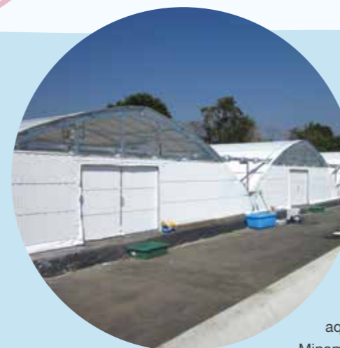
▲ Shirahime shrimp-rearing tank covered by a greenhouse to maintain the breeding water temperature
