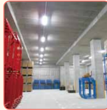
Inside a refrigeration room with good space for cargo
