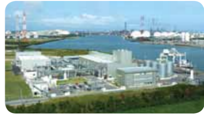
Aerial view of Kashima Plant
