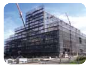
Kashima Pharmaceutical Plant under construction on adjoining land
