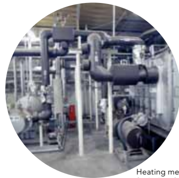
Heating medium boilers which can be fueled by fish oils after distillation
